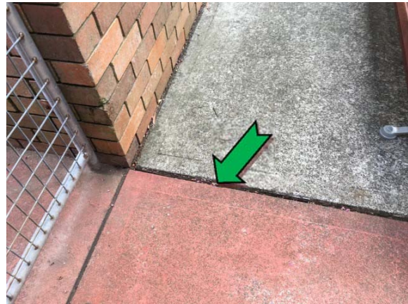
Photo 4. Exterior, throughout, floor, expansion joints – non asbestos-containing construction mastic.
